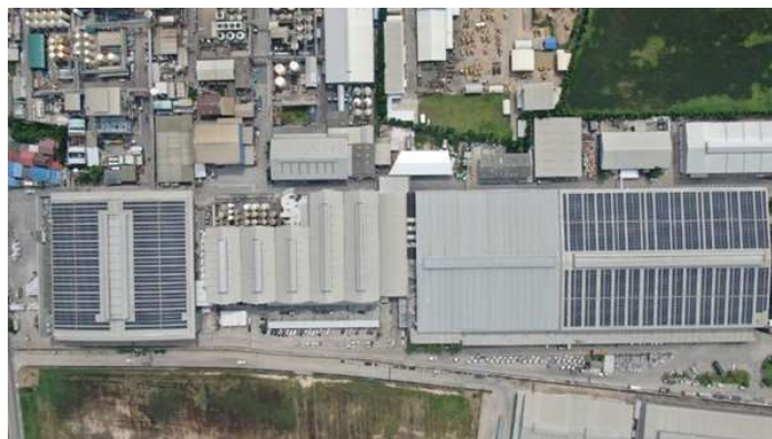
Solar Rooftop at Warehouse 2 and Store 2
